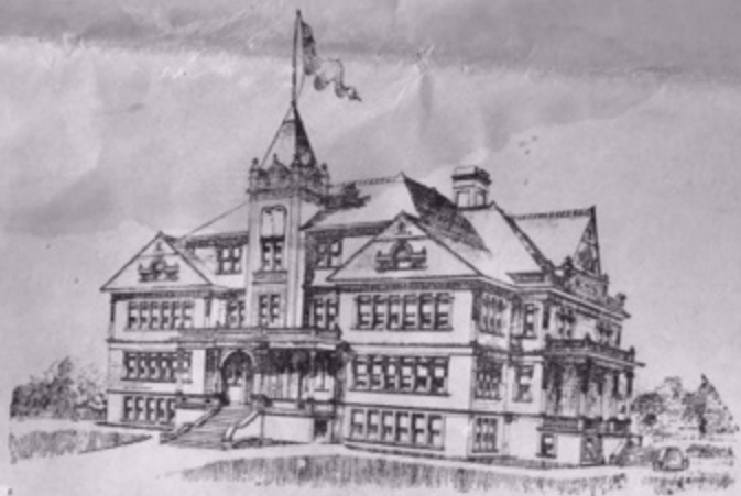
NORTH SCHOOL BUILDING.
