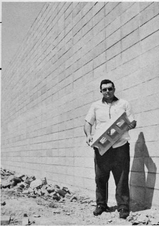
Lyman Bennett is holding one of the expanded shale blocks used in the construction of the new building. These blocks are available now from the Basalt Rock Company, HOWard 4-7619. Plant is locted one-half mile south of French Camp on Highway 50.
