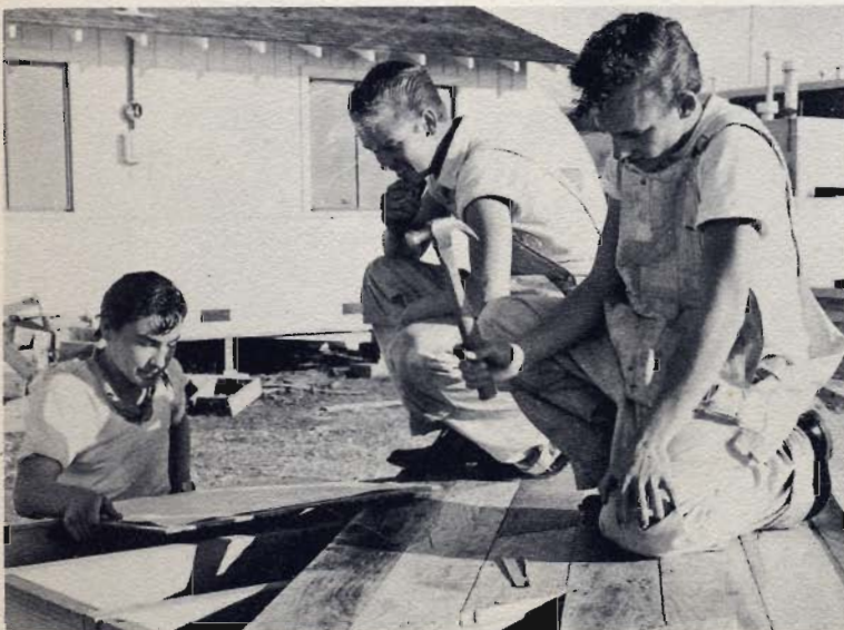
Carpenter trainees laid subflooring.
