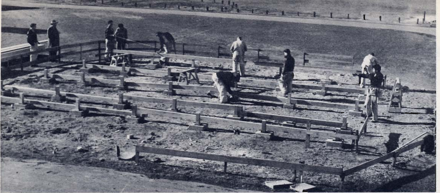
House in its early stages.
