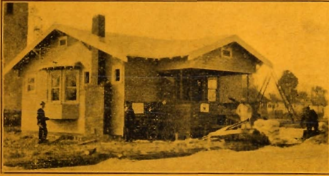
ONE OF OUR HOUSES IN COURSE OF CONSTRUCTION
