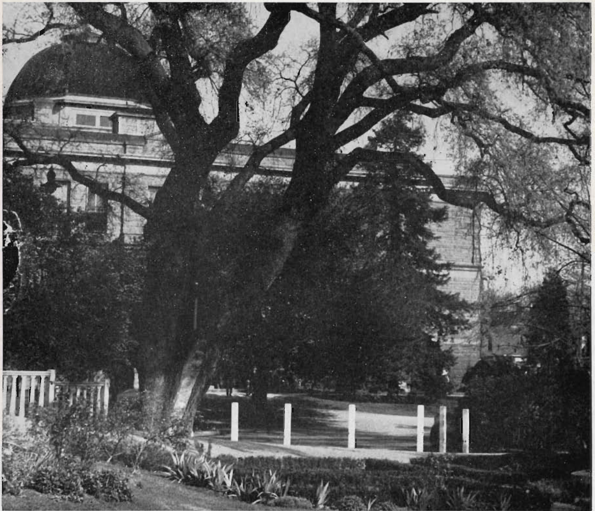
West side main building and west glade looking from front of auditorium
