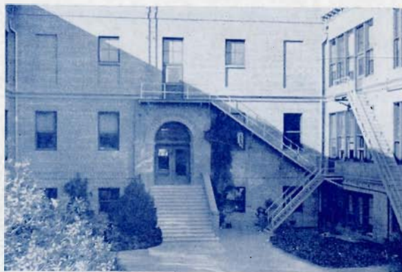
Courtyard Between Commercial and Science Building
