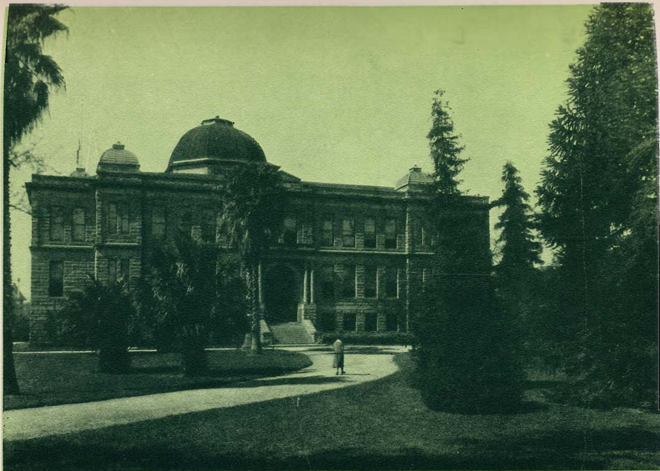
EAST VIEW OF THE CAMPUS
