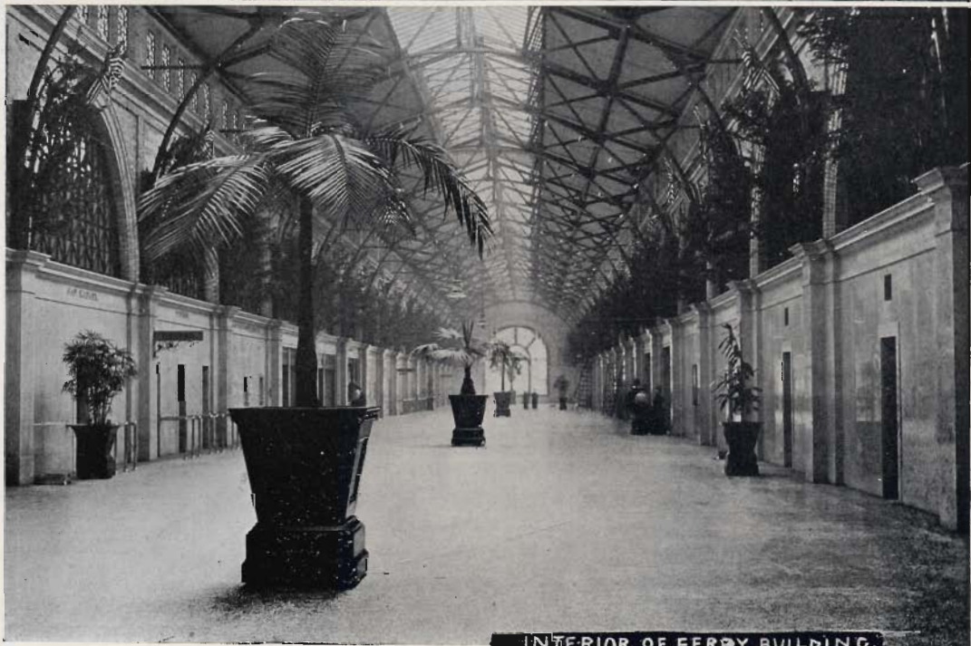
INTERIOR OF FERRY BUILDING.
