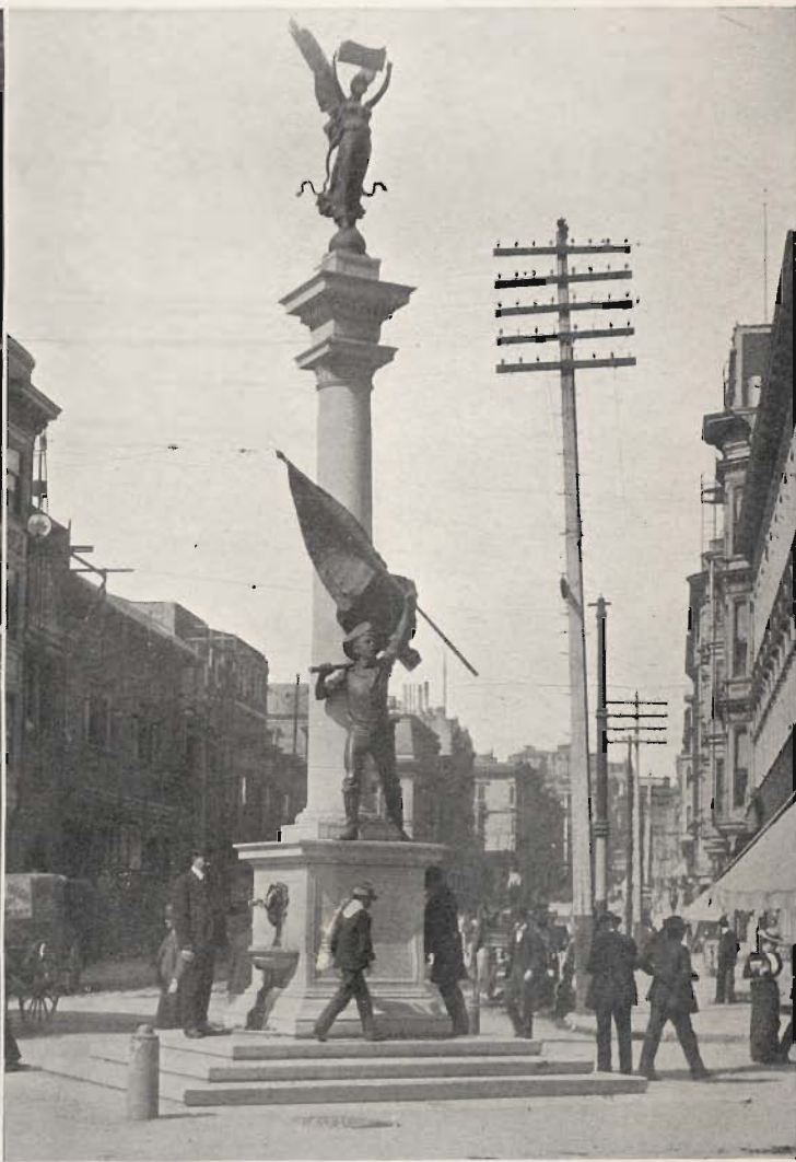
NATIVE SONS' MONUMENT Corner Mason, Turk and Market streets.
