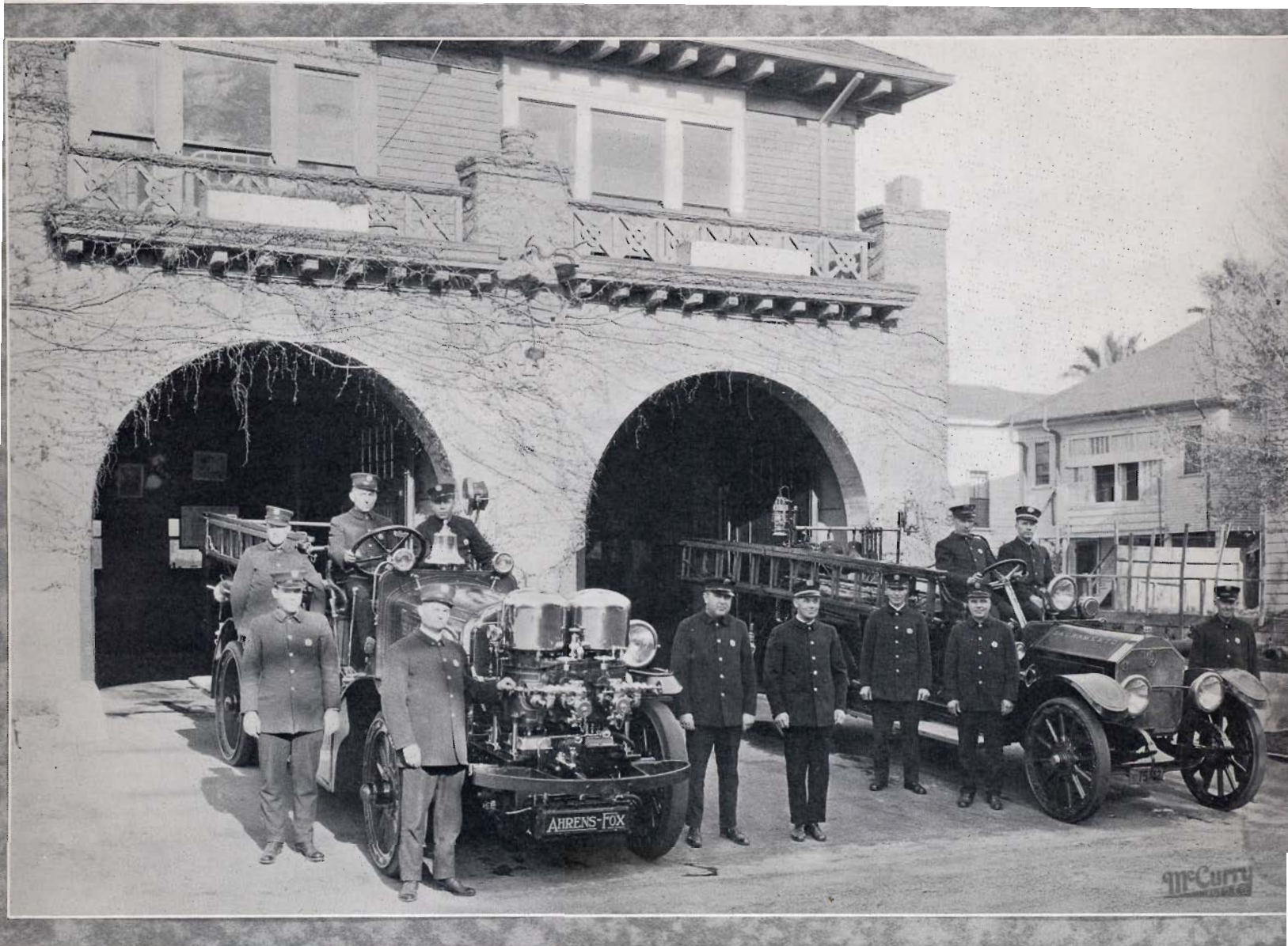
Engine Company No. 4—1214 26th Street
