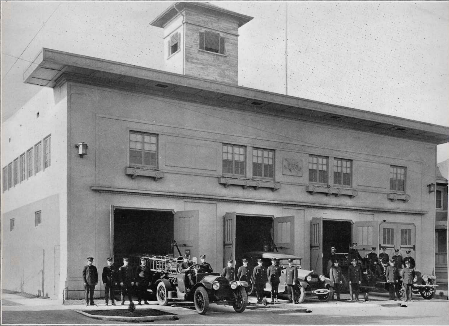
Engine Company No. 6 and Truck No. 3—4th Avenue, 34th and 35th Streets
