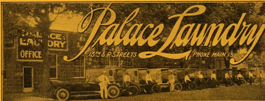
A. O. (Jack) JOHNSON, The Practical Laundryman
