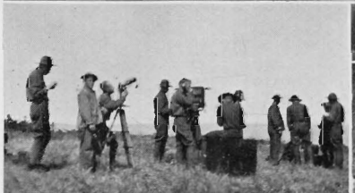
Looking for enemy aircraft—locating instruments on the 3-inch AA. Battery.
