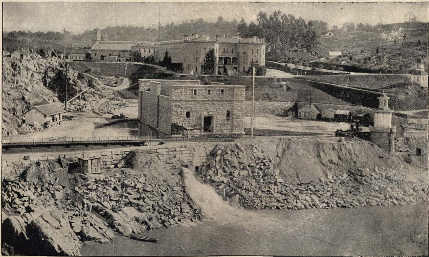
STATE PRISON AND POWER HOUSE, FOLSOM, SACRAMENTO COUNTY, CALIFORNIA.
