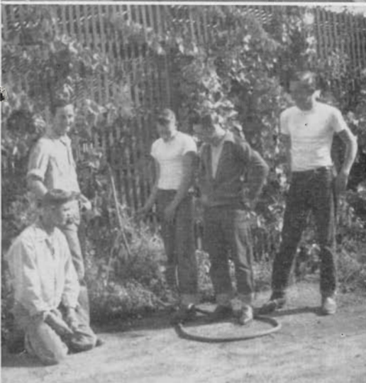
C. Rockholt, J. Tilden, J. Livingston, O. Fox, and D. Fricke begin to build cement walk behind Jr. High. O. Fox, N. Thompson, C. Rockholt, J. Tilden, C. Arnold, F. J. Robbins and A. Gutierrez finish the job. Bottom: Officers were O. Fox, B. Thomson, E. Berry, L. Lady and D. Todd.
