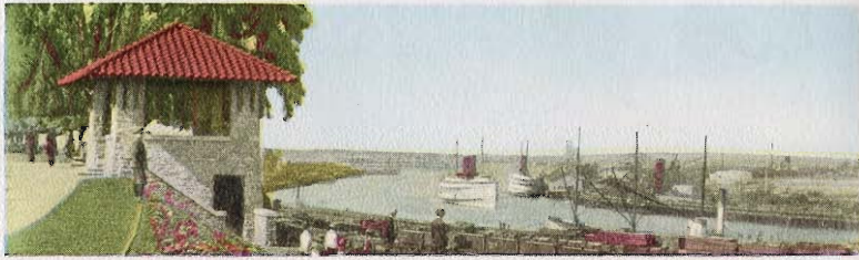
Portion of Los Angeles Inner Harbor
