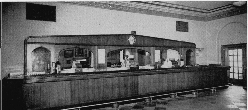
The Bar. (Door at extreme right opens to small sun deck)
