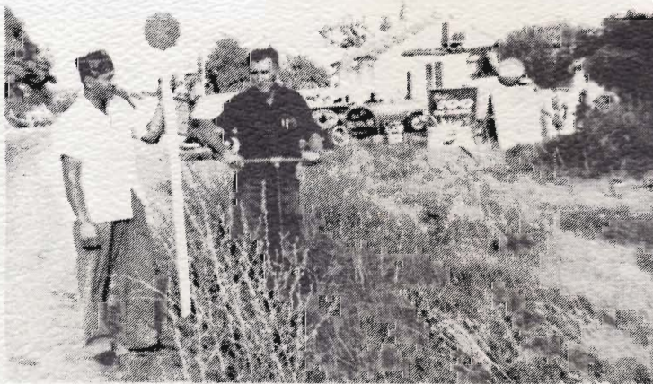
Comm. Charles Renfroe digs hole for installation of a DRIVE CAREFULLY sign on south side of Sylvan School, while Joe Giusti assists. In back ground is the old Bruce Williams service station and bar, now the site of a franchised chicken store.
