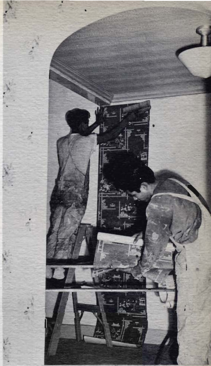
wall paper room --- part of paint shop
